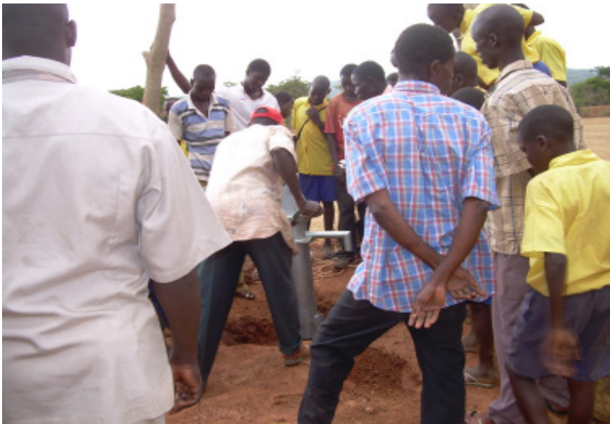
Fixing of the water pump at Nabuganda
