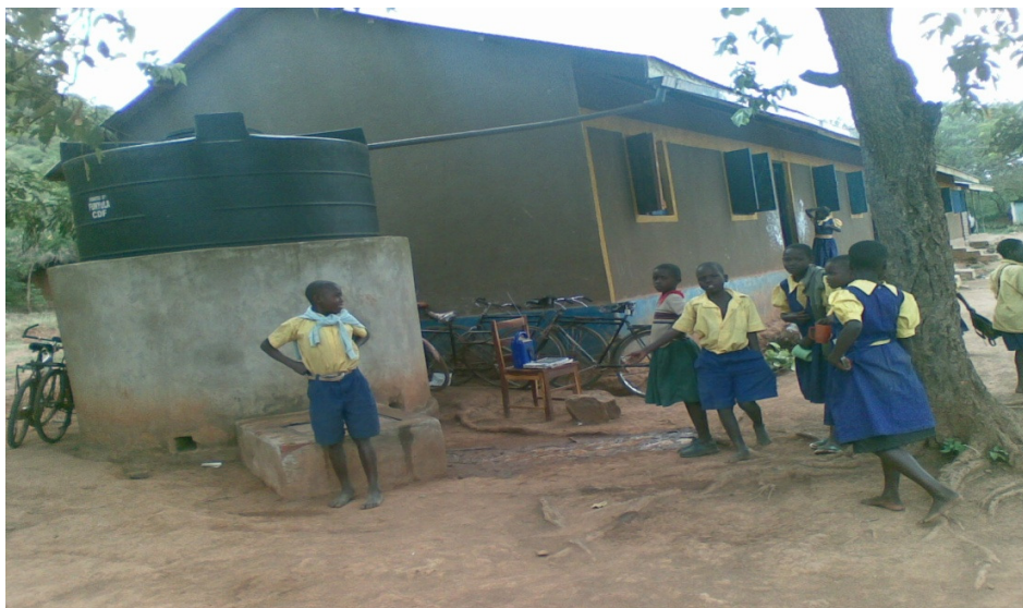
The water tank in the above photo is one of the tanks donated to the schools in Busia by the ministry of education. Small in size and cannot store enough water for use. Water is usually used by the teachers and cooking meals for the students. Rainfall is seasonal.
